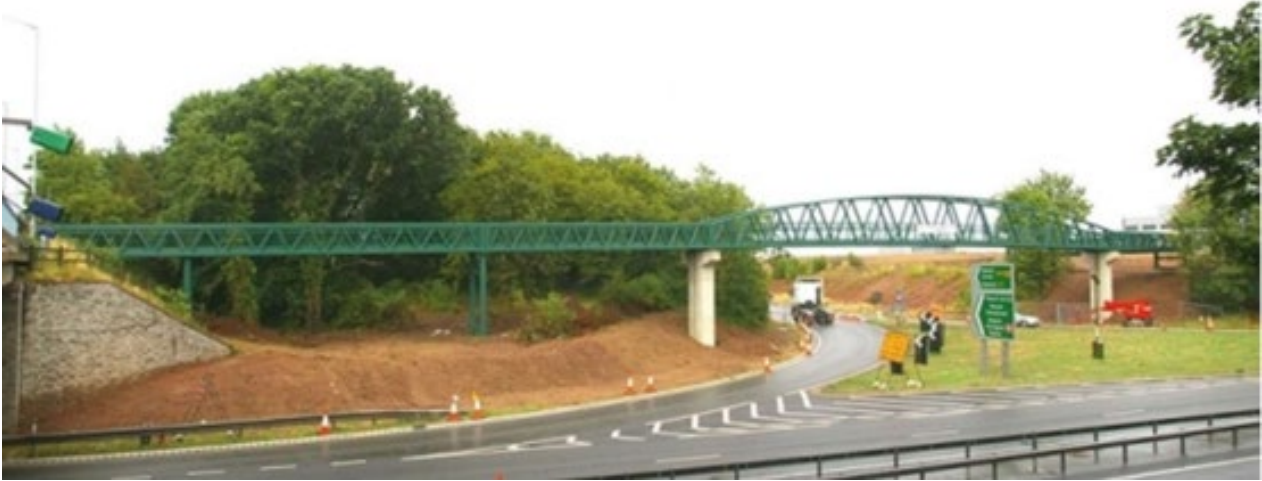
Image 3.9: Example of multi span through truss footbridge structure
