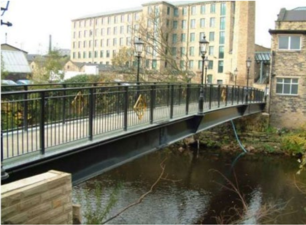
Image 3.16: Steel edge beam bridge
