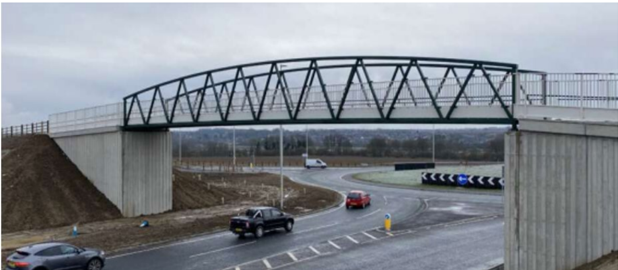
Image 3.10: Example of shorter span steel through truss over road
